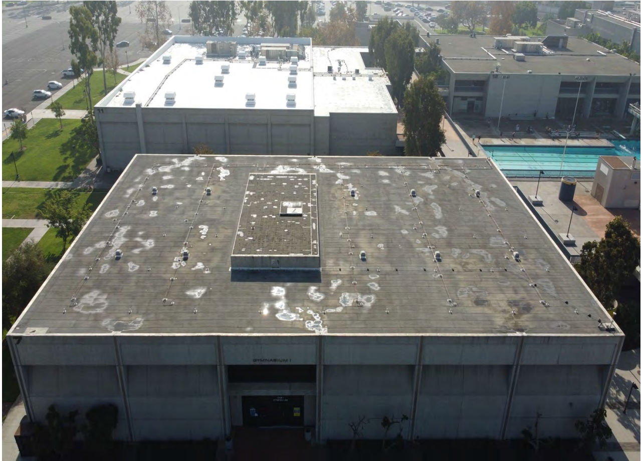
Building 7, Gym I for Cypress College has a flat roof that appears to be the original built up roof that was installed when the building was built.
