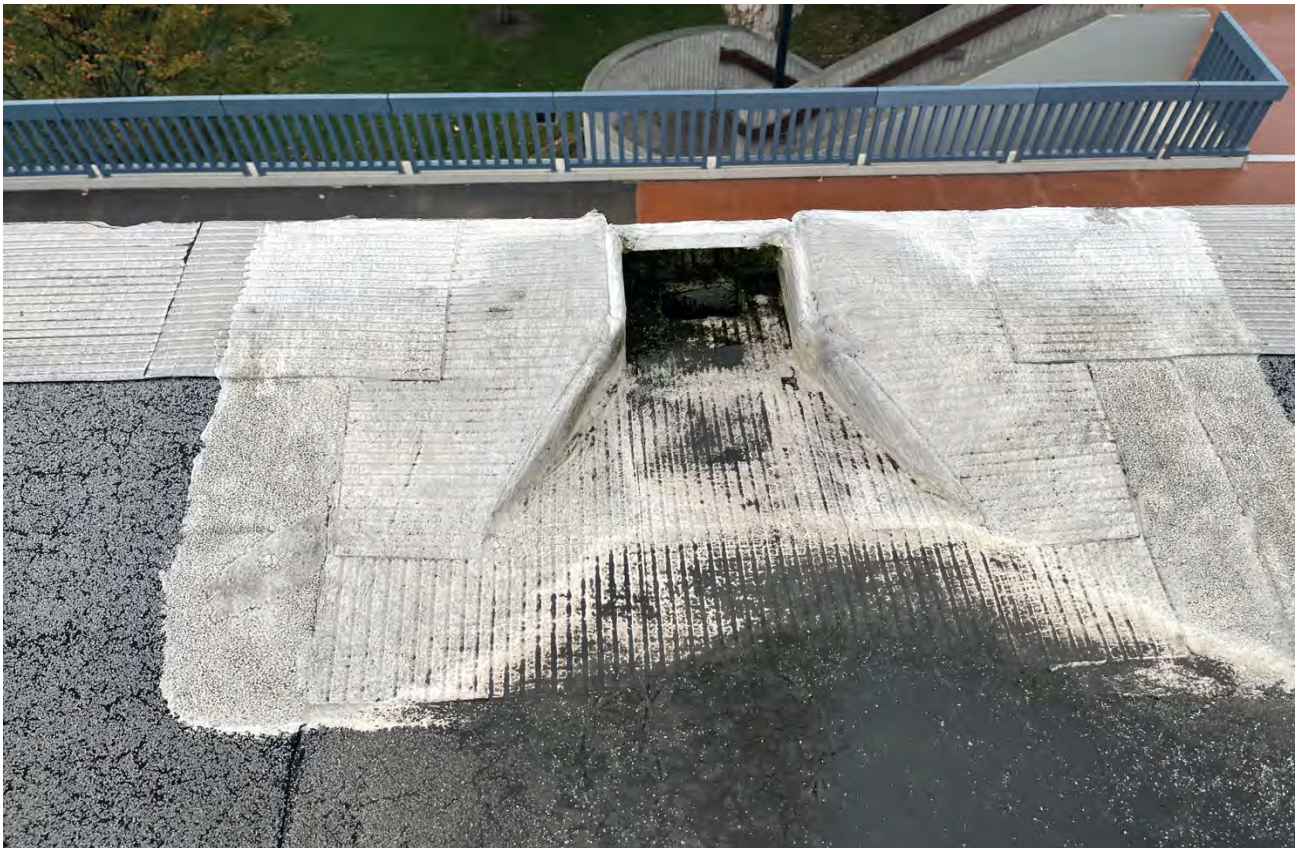
The roof drains to scuppers along the perimeter of the building. It is recommended that these scuppers be encapsulated during roof work and WeatherWeld to be applied to the outside edge of the parapet wall per spec,
