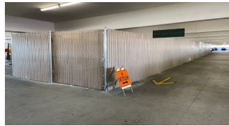
Swing Space — New M&O [Construction]
