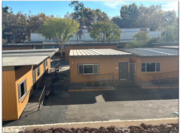
Swing Space / Interim Housing—Modular Building Construction Activities
