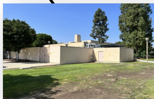
Wilshire Chiller Plant Relocation [DSA Review]
