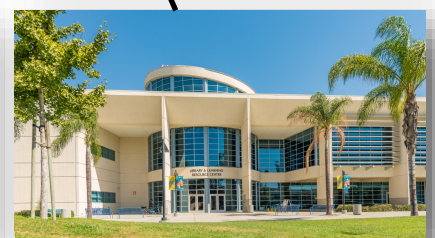
LLRC Secondary Data Center (Phase II) [ Implementation ]
