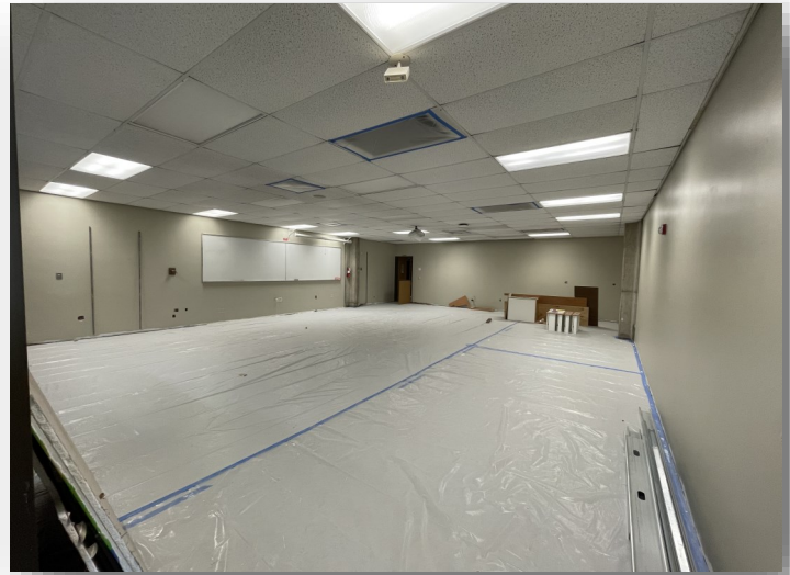
Swing Space—Fine Arts—Construction Activities
