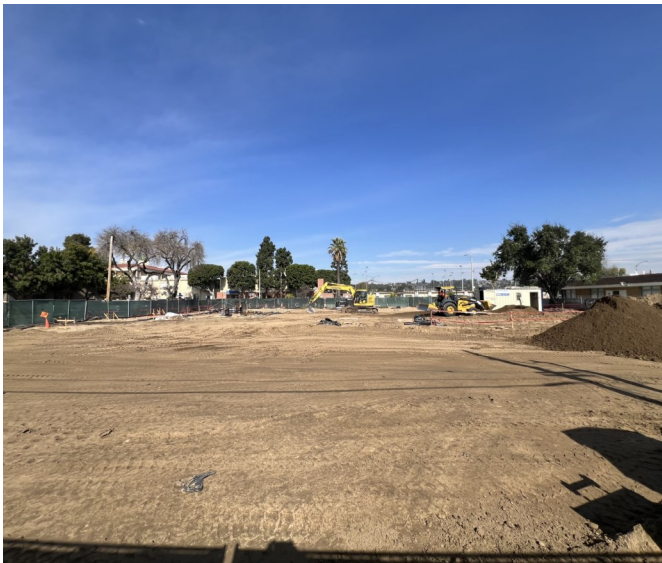
Chapman / Newell Instructional Building -- Construction Activities
