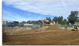
New Maintenance & Operations Building [Construction]
