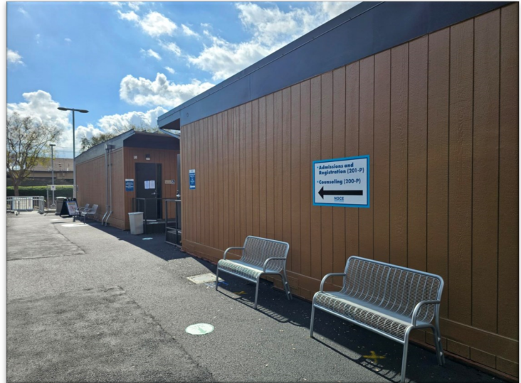
Swing Space—Interim Housing—Completed Construction
