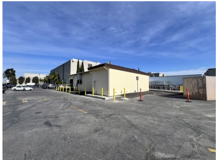
Swing Space—Hotel, Restaurant, and Culinary Arts: Kitchen, and Restroom and Dining Room—Modular Construction Activities
