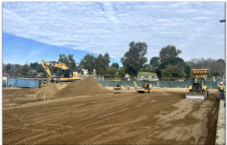
New M&O Building - Construction Activities
