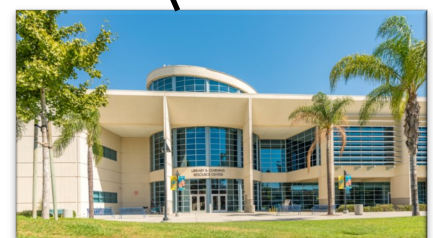
LLRC Secondary Data Center (Phase II) [Close-Out]
