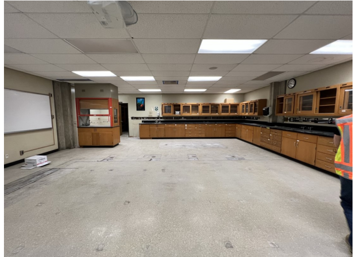
Swing Space—Fine Arts—Construction Activities
