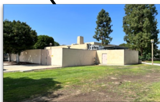
Wilshire Chiller Plant Relocation [DSA Review]
