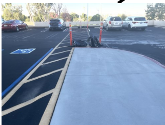
Anaheim Campus Tower First Floor Life/Safety Renovation [DSA Review]
