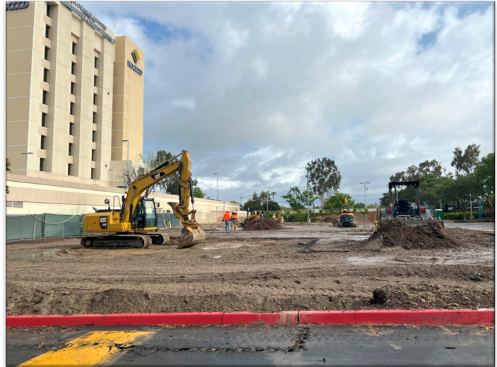
Swing Space / Interim Housing—Demolition of the Playground
