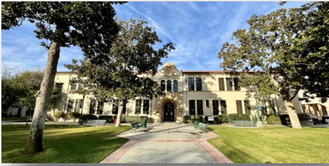
Renovate Building 300 [Planning]
