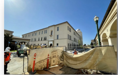
New Instructional Building [Construction]
