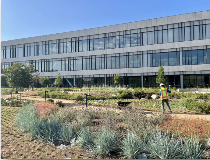
New SEM Construction Progress — August 2021
