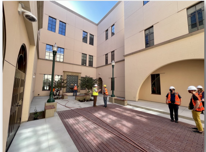
New Instructional Building Construction Progress —August 2021
