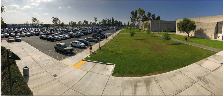
Completed Parking Lot 5 Realignment from the Library & Learning Resource Center (LLRC) at Cypress College
