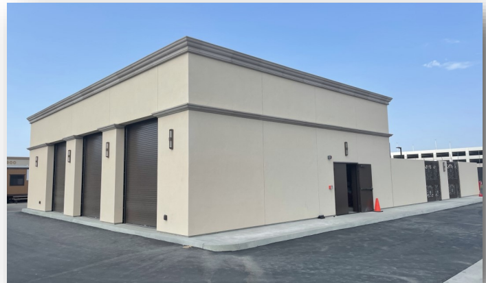
Central Plant Construction Progress — August 2021
