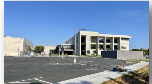
New Science, Engineering and Mathematics Building [Construction]
