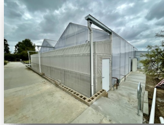
Greenhouse Replacement [Close-out]
