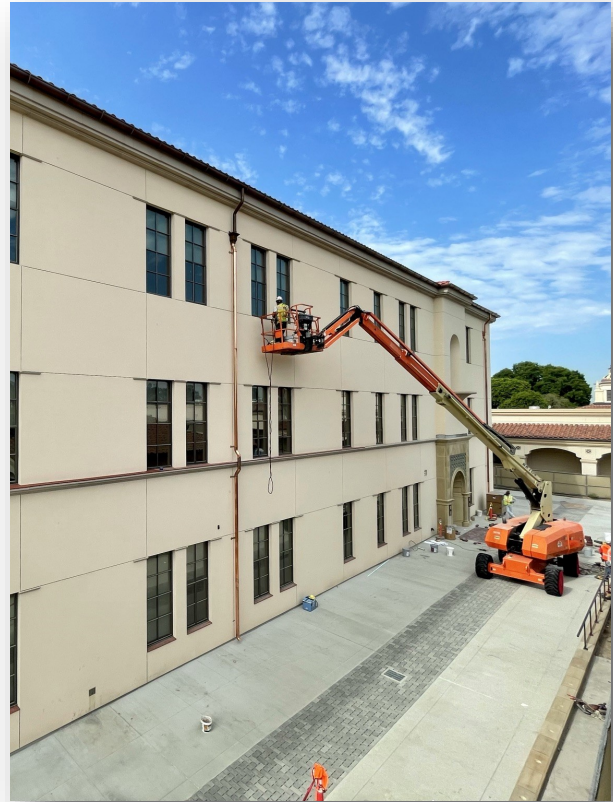
New Instructional Building Construction Progress — August 2021
