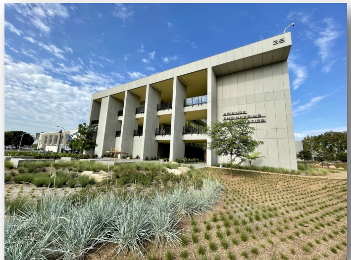
New SEM Construction Progress — August 2021
