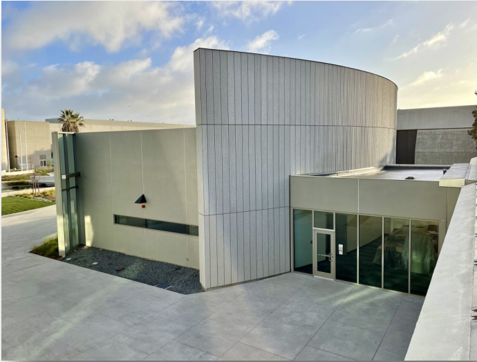
VRC and Pond Construction Progress — February 2021
