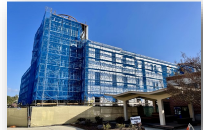
New Instructional Building [Construction]
