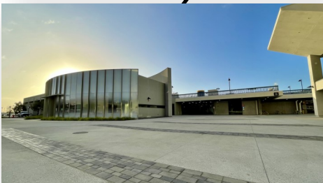
New Veterans' Resource Center & Student Activities Center Expansion [Construction]
