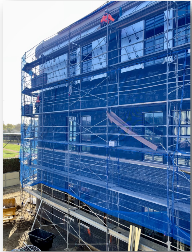
New Instructional Building Construction Progress —February 2021
