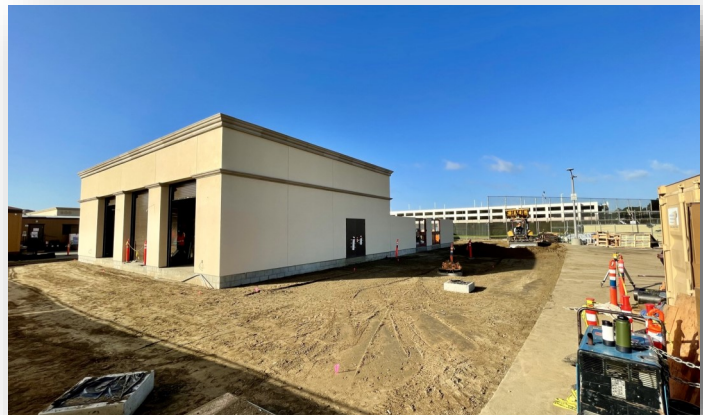
Central Plant Construction Progress —February 2021
