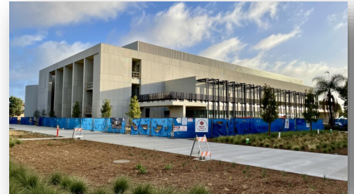
New Science, Engineering and Mathematics Building [Construction]
