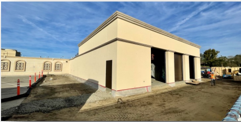
Central Plant Replacement and Expansion [Construction]
