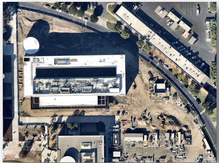
New SEM Aerial Construction Progress —February 2021
