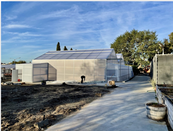
Greenhouse Replacement Construction Progress —February 2021
