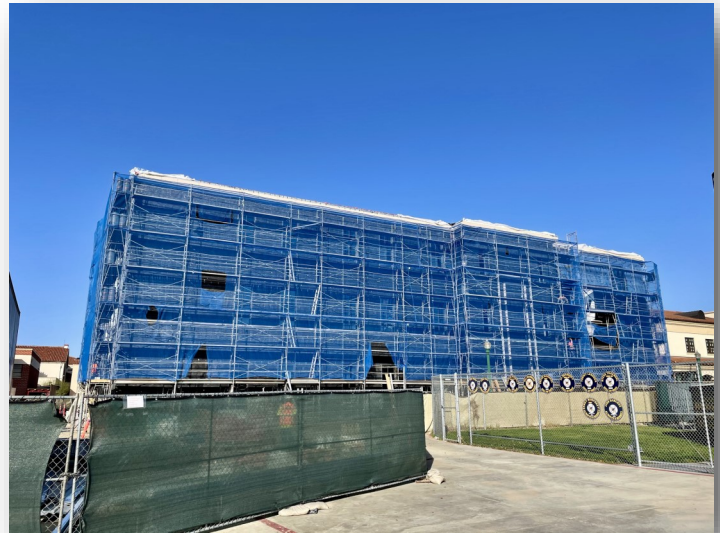
New Instructional Building Construction Progress — February 2021
