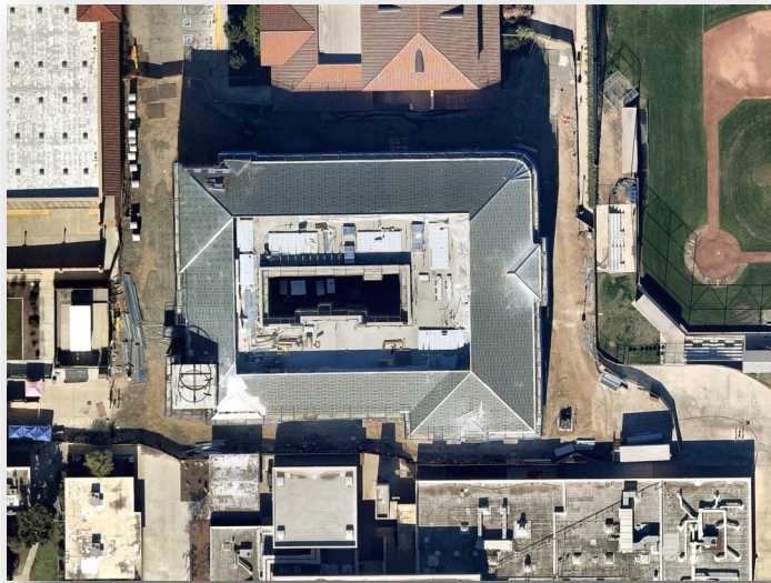
New Instructional Building Aerial Construction Progress —February 2021
