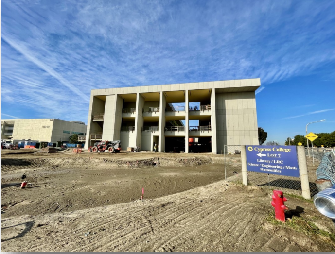
New SEM Construction Progress — February 2021
