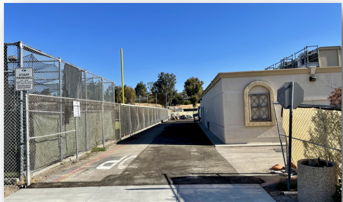
Central Plant Construction Progress —April 2021
