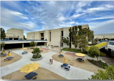
Fine Arts Building Renovation [Design - Design Development]
