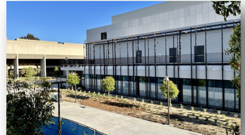
New Science, Engineering and Mathematics Building [Construction]
