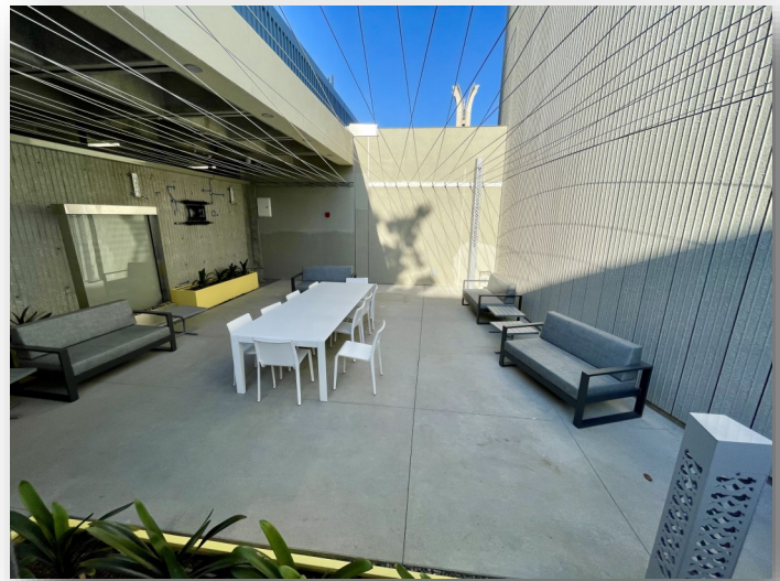
VRC Exterior Courtyard Construction Progress —April 2021
