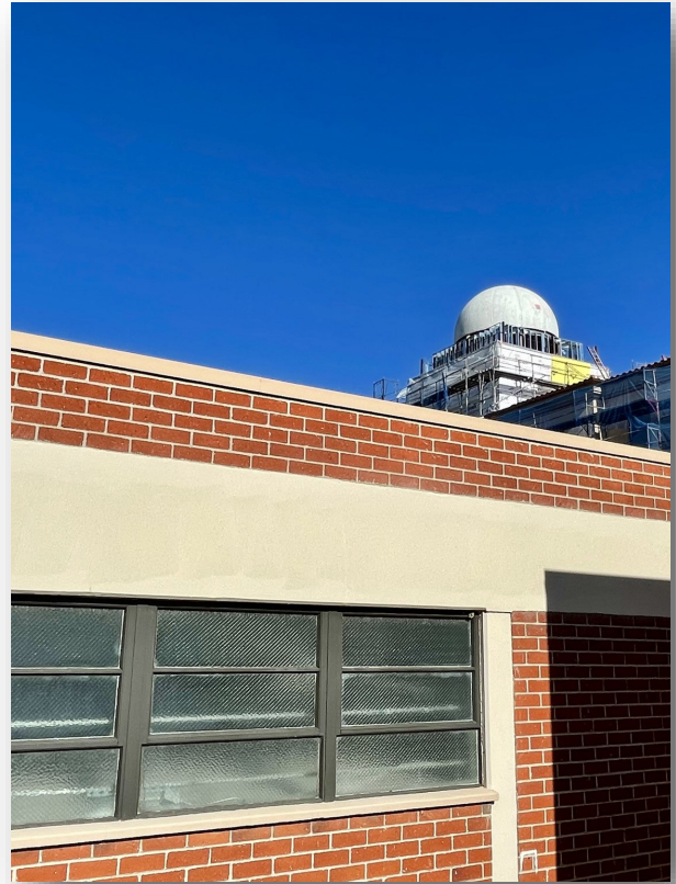
New Instructional Building Construction Progress —April 2021
