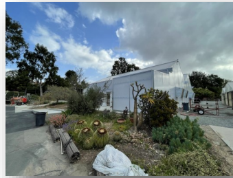
Greenhouse Replacement [Close-out]
