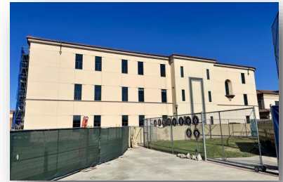
New Instructional Building [Construction]
