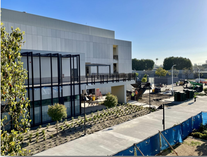
New SEM Construction Progress —April 2021
