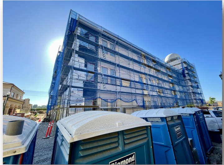
New Instructional Building Construction Progress —April 2021
