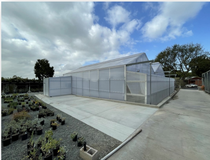
Greenhouse Replacement Construction Progress — April 2021
