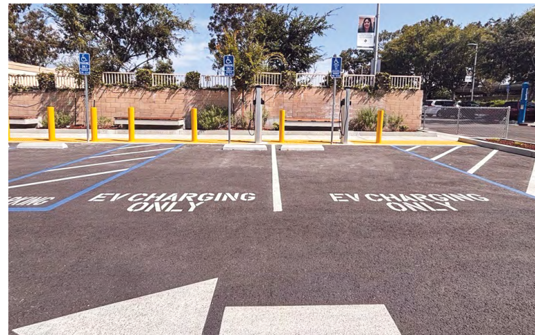
Completed Lot and Installed EV Charging Stations – Restore East Parking Lot – Anaheim Campus
