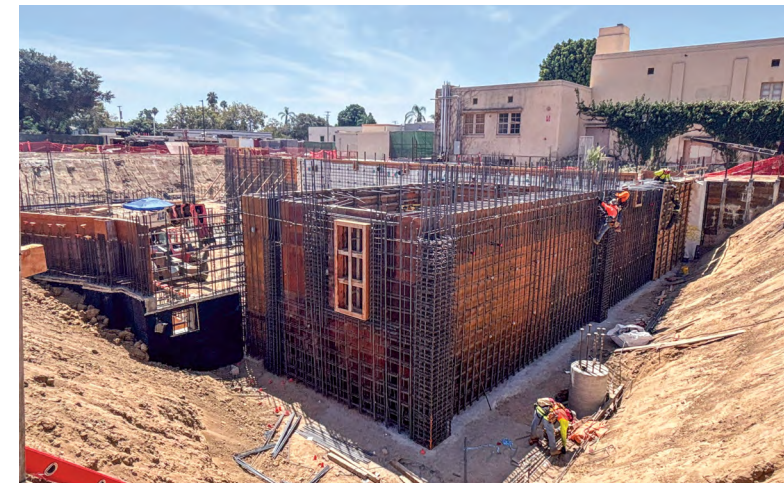
Auditorium Basement Construction – New Performing Arts Complex – Fullerton Campus
