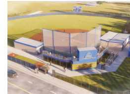
Softball Field Renovation [Design-Construction Documents]
