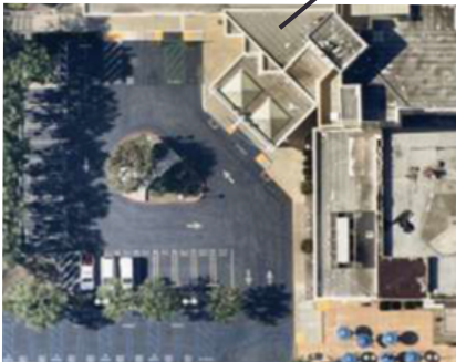
Exterior Green Community Space Enhancement [Construction]
