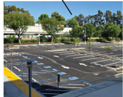
Restore East Parking Lot [Close-Out]
