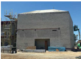
New Performing Arts Complex - Demolish Buildings 1100 & 1300 [Construction]
