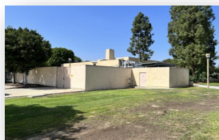
Wilshire Chiller Plant Relocation [Design—Construction Documents]
